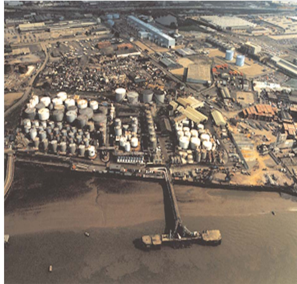
Dagenham Dock as it is now
